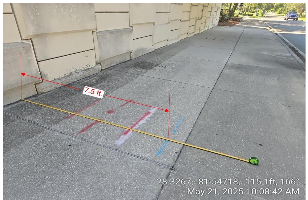
Underground 16-inch diameter water main is 7.5 feet away from proposed piling activity at the MCE wall
